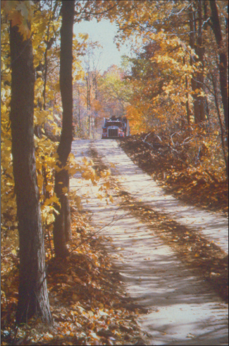
Figure 2. Well-designed and maintained haul road.
