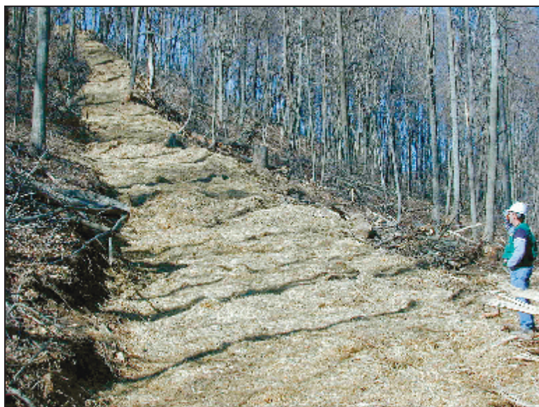
Figure 27. Properly installed mulch on new seeding.
